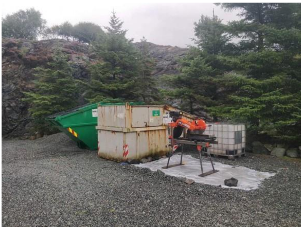
Figure 3-7: Core cutting area
