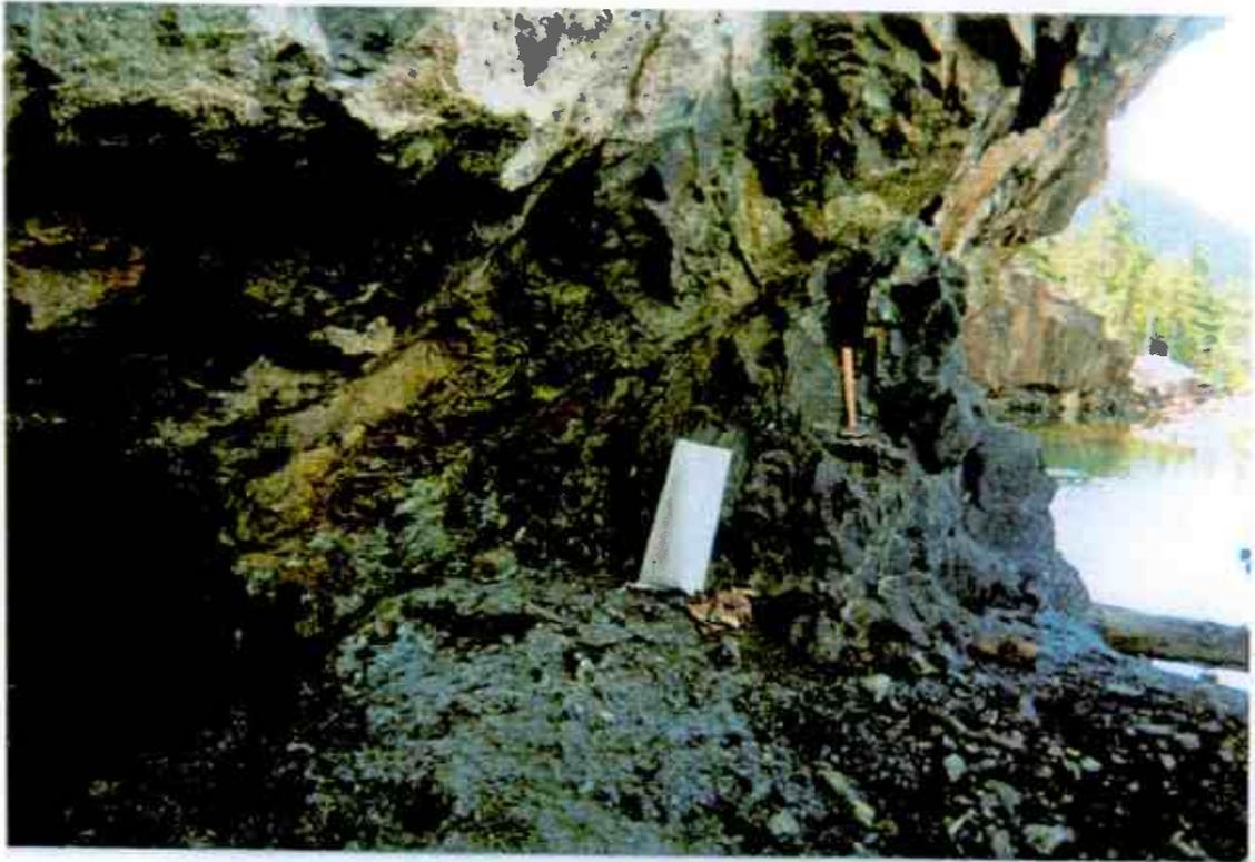
Figure 19: Photo of a pillar supporting the hanging wall at Bø Mine
