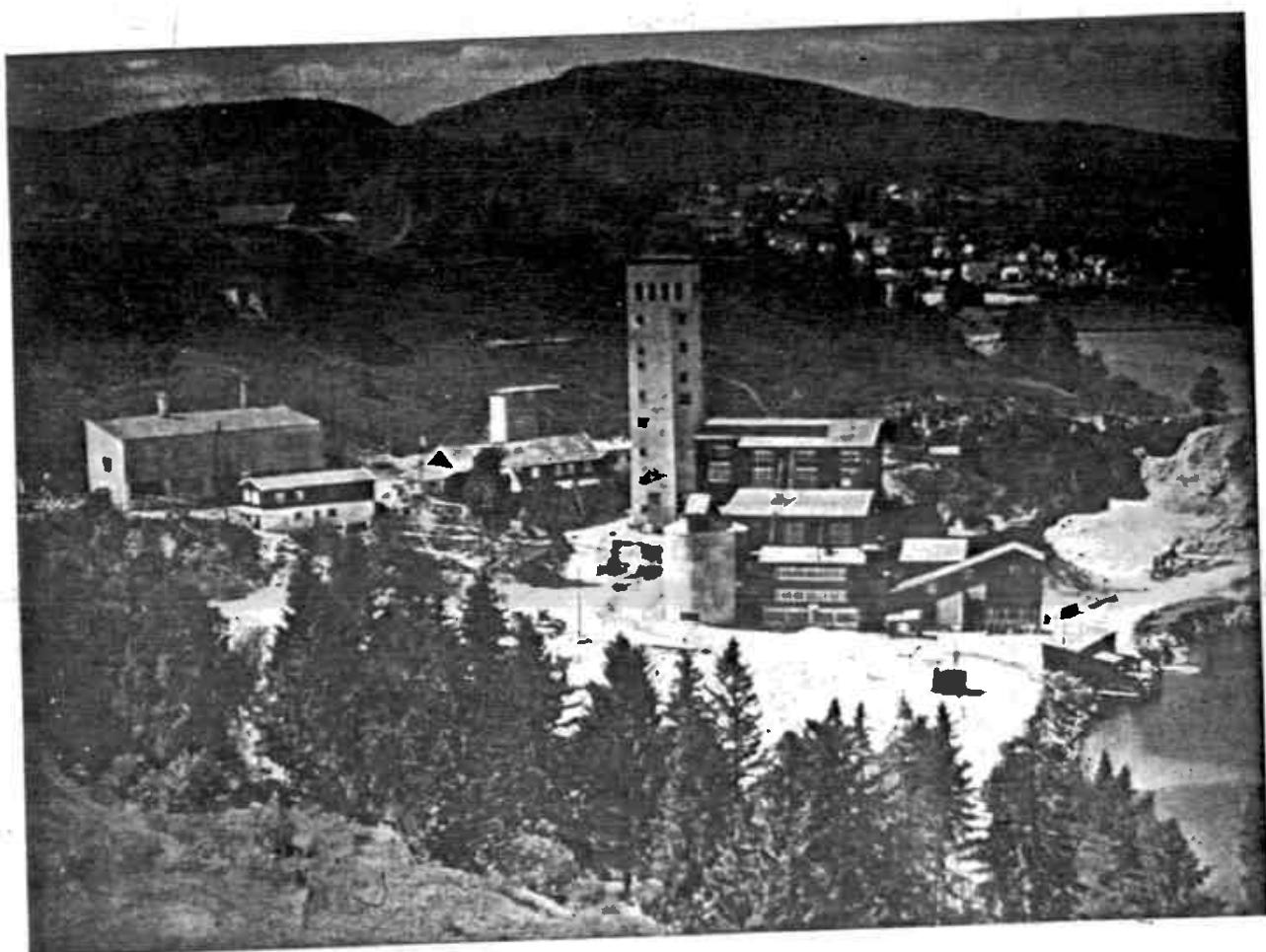
FIGURE 1. 1950'S PHOTO OF NORSK BERGVERK'S MINE FACILITIES WITH HEADFRAME FOR 270M SHAFT. ALSO SHOWN ARE MILLING AND ORE DRESSING PLANTS FOR PROCESSING PYROCHLORE MINERALIZATION.
